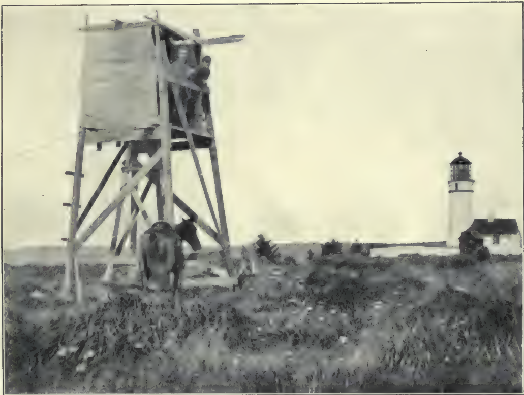
FIG. 4.—STATION CAPE SHOWING THE OBSERVING TOWER WITH THE WIND SHIELD.
